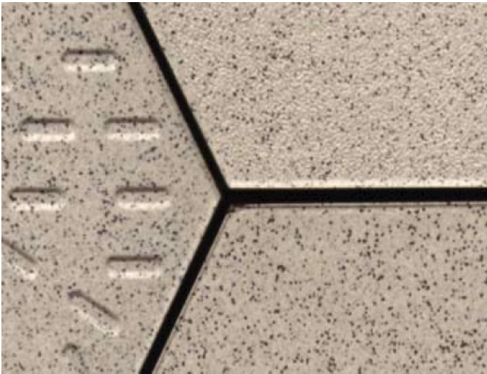
2. Hexagonal, Carolina Clay, fully-vitrified TUFCEM tiles used at BI Chemicals
